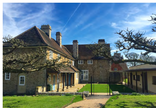
ST BENEDICT'S CENTRE, WEST MALLING
